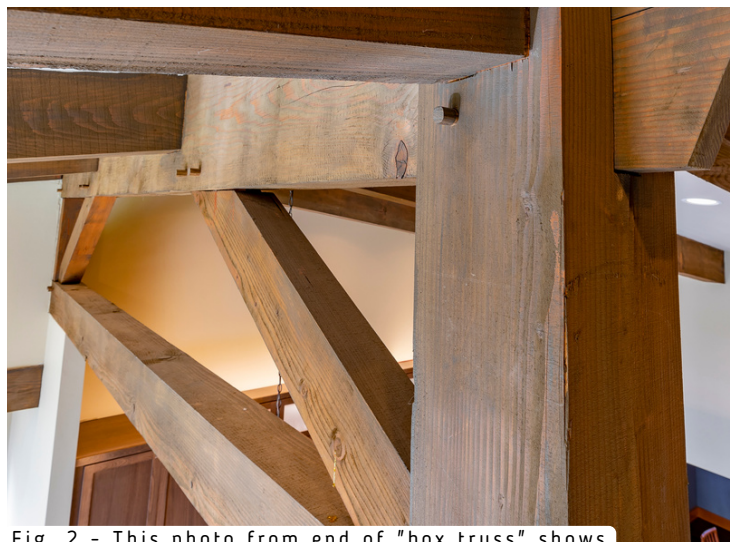
Fig. 2 - This photo from end of "box truss" shows typical geometry and thru tenon. (Top right corner.)
