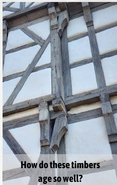
Old Fachwerk(half-timbered) city apartments in Erfurt with exposed lateral bracing.
